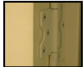
Hinge spacer installed
