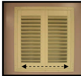
RACK the bottom of your frame to the left or right for an even reveal.
