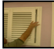
Insert panel into position.
