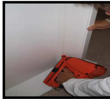
**Note: After ensuring that your center stiles and side boxout are aligned, you can go back and add additional nails/screws to completely secure your boxout frame.**
