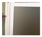
Using a level, ensure the frame is plumb (straight up and down) and temporarily secure to the opening with a screw/nail at the top and bottom of the frame. Use shims if necessary to keep frame plumb.
