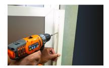
Close panel against the non-hinged frame and check to see there is approximately a 1/8" even space between the panel and frame. Adjust as necessary to achieve even spacing.
